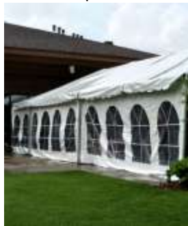
Installation of Tent Sides | $75
